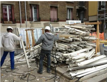
Dismantling of windows.
