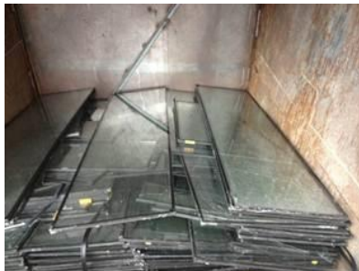
Stacking the window in skip.
