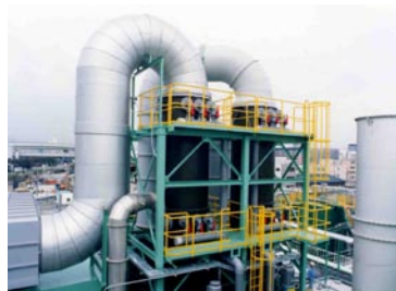
Odor control device for rendering plant
